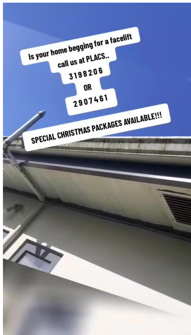
Roofline and guttering
