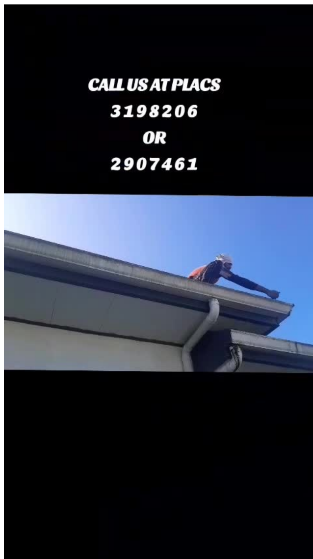
Roof cleaning in progress
